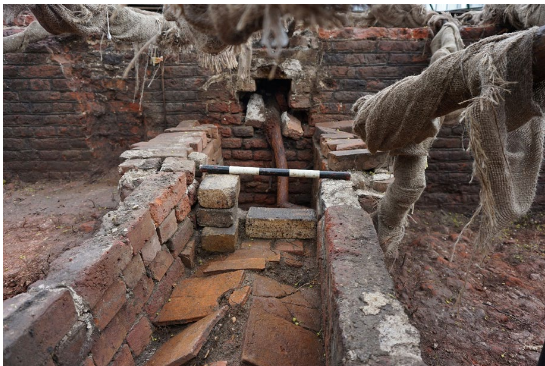
Fig 15: Photo of root disturbance through an area of weakness at Hampton Court Palace, London (©Oxford Archaeology)
