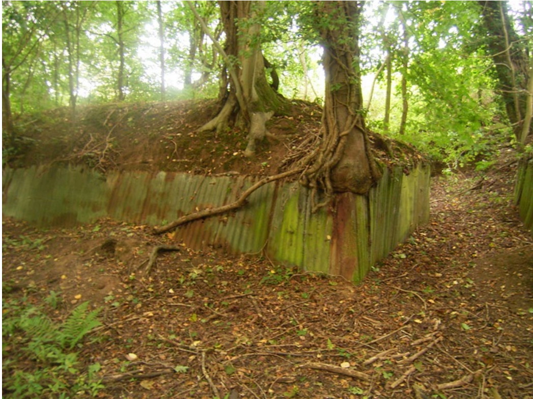
Fig 33: Root-affected historic building/structure at Chilworth Gunpowder Mill (©Oxford Archaeology)
